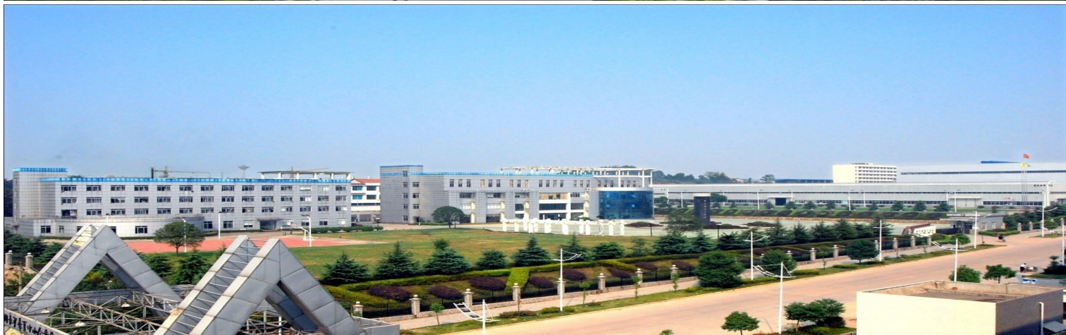
Truking Phase-I manufacturing base(2002)
